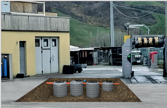
Installation de station de lavage
